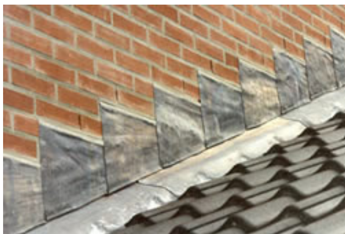
Figure 1 Lead flashing used at a wall-roof transition [4].
